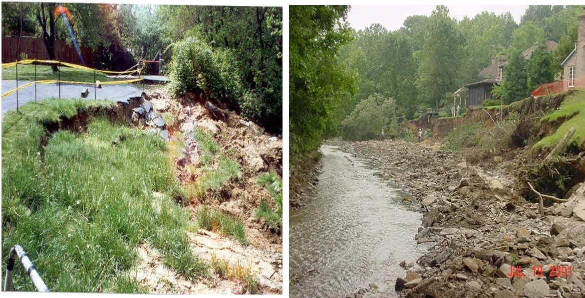
Landslides Triggered by Erosion
